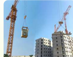
Light House Project MOHUA, Ranchi
