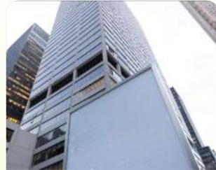
Lumina CloudInfra Data Center, Mumbai
