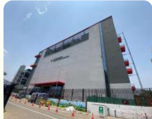
STT GDC Data Center, Pune
