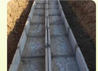
L&T Cable Trenches, Gujarat
